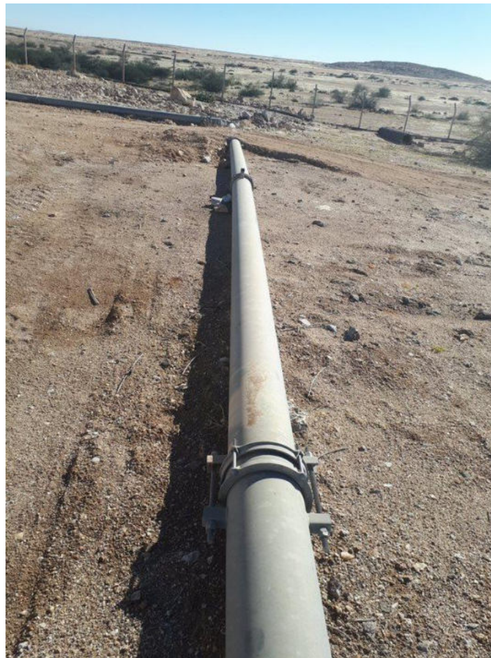
Figure 5: 250 mm dia. quick coupling steel pipes with clamps
