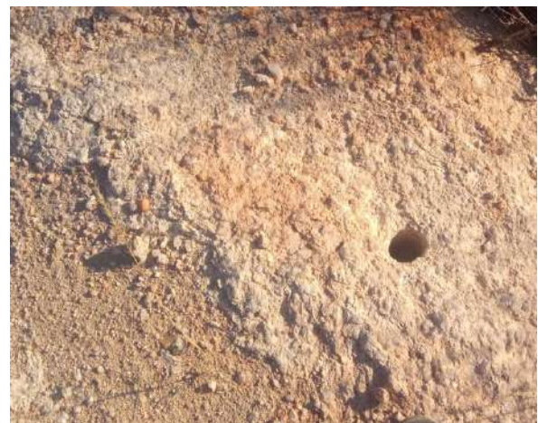
Photo 20: A drilled blast hole on the Rock Face
