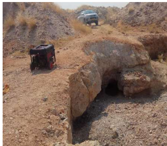
Photo 4: A Portable Generator
