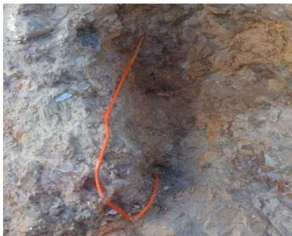
Photo 19: A charged blast hole with live fuse
