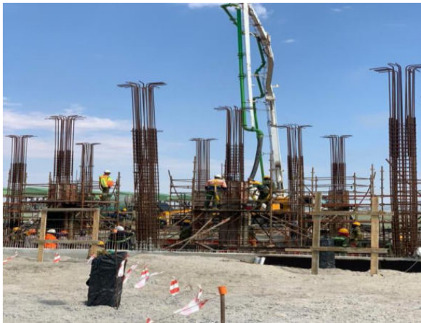
Picture 3: Progress on the Workshop
