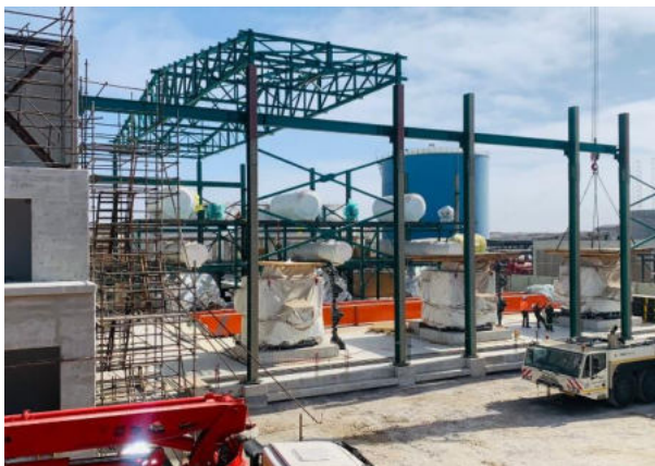
Picture 5: Progress on the Powerhouse and installations
