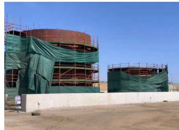
Picture 6: Progress on the Tank farm
