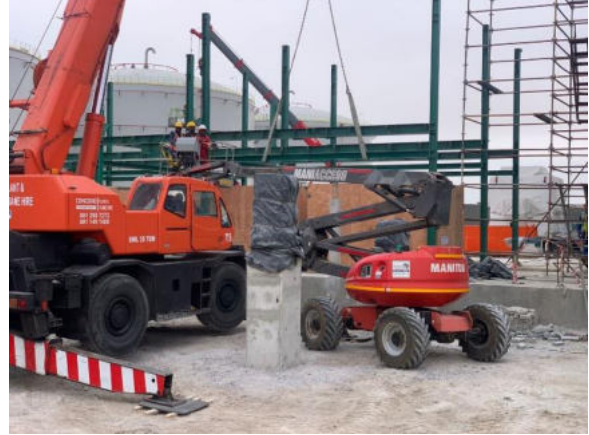
Picture 2: Crane operation on-site
