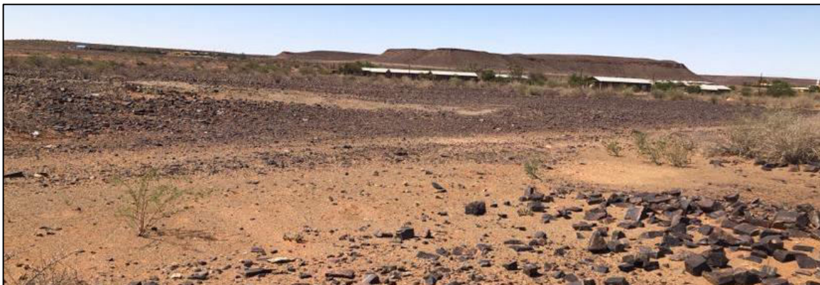
Figure 16: Buildings next to the Project Site
