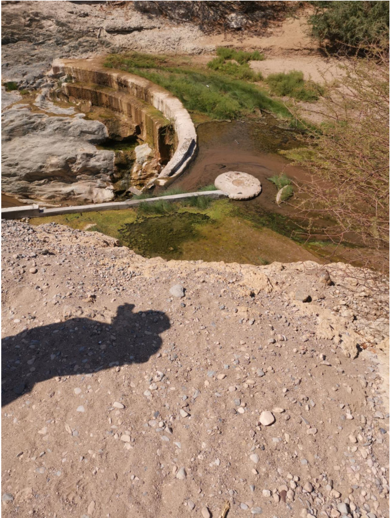
Figure 5 Fountain where the project will draw water for irrigation
