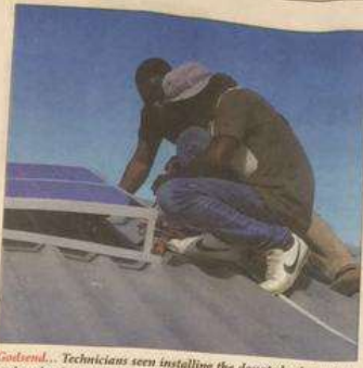
Godsend... Technicians seen installing the donated solar system at the school
