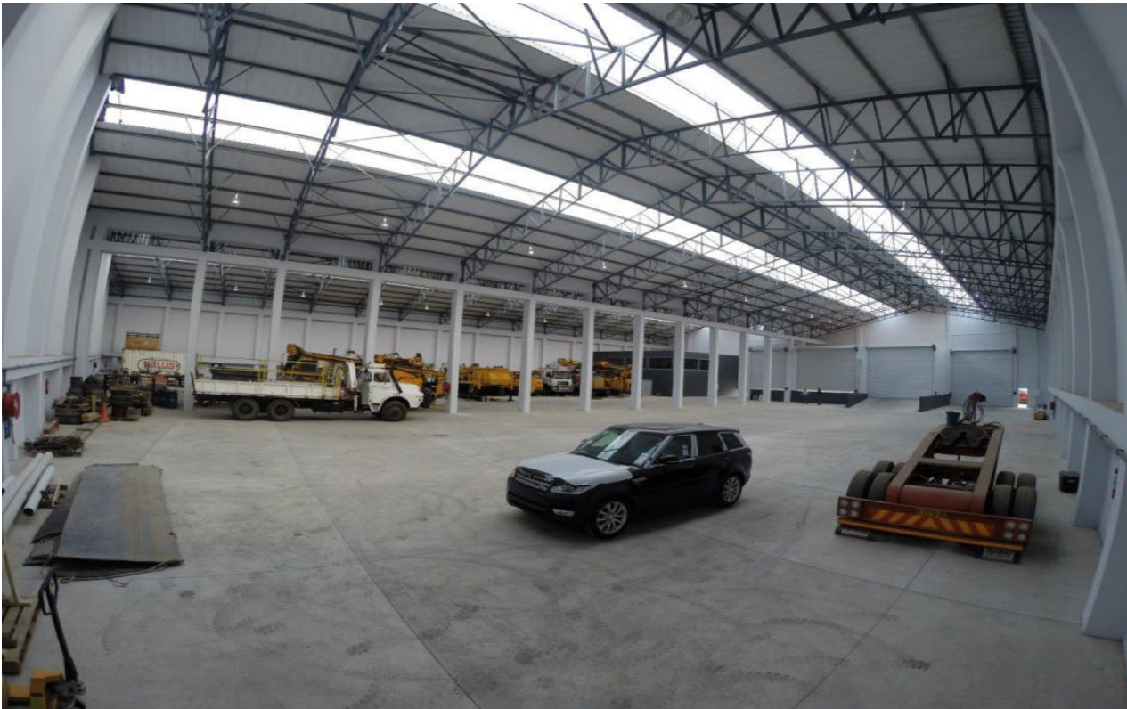
Figure 8: Inside View of the Warehouse Taken from The Eastern Angle
