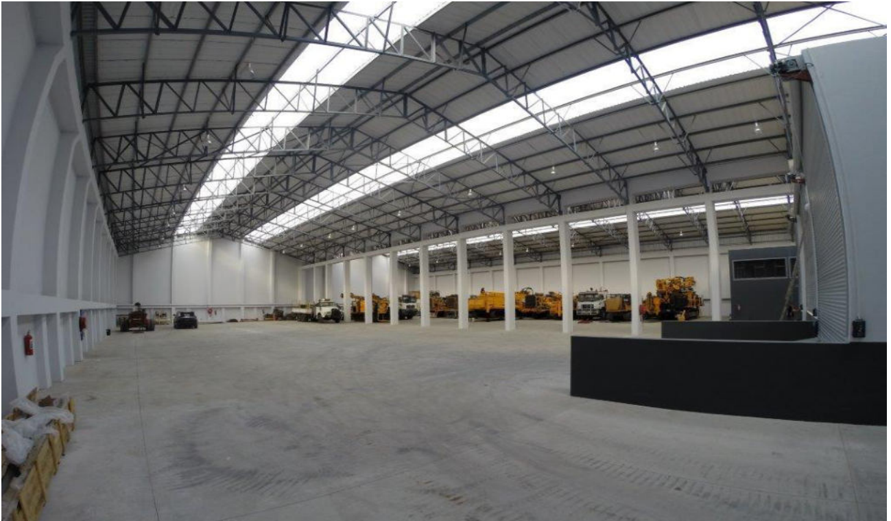
Figure 11: From the eastern side, a panoramic picture of the Warehouse (interior)
