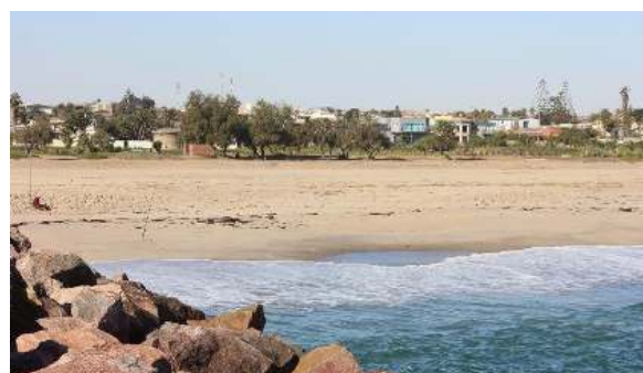
Photo 25. Cable landing area
