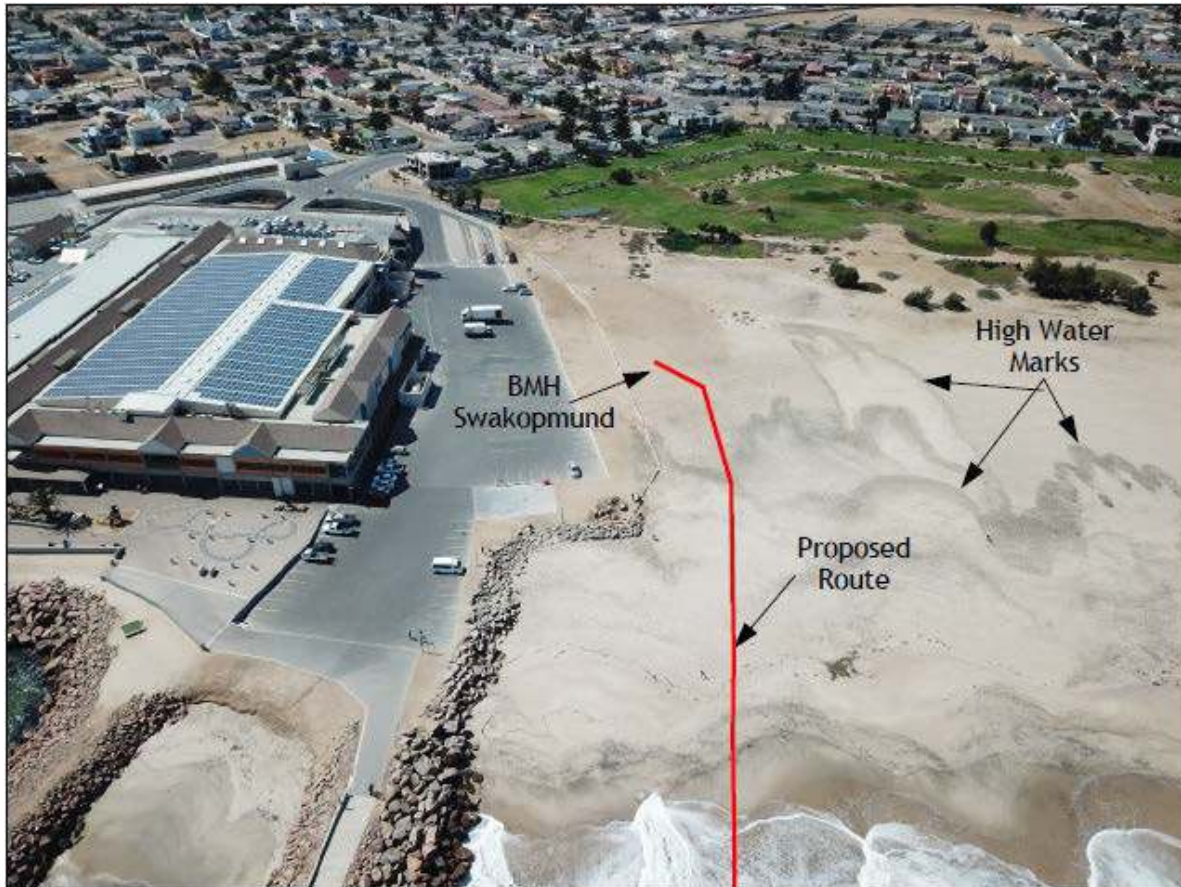
Figure 10 View of the proposed route to the BMH south of the mall at Swakopmund and Paddock Garden inland of the BMH
