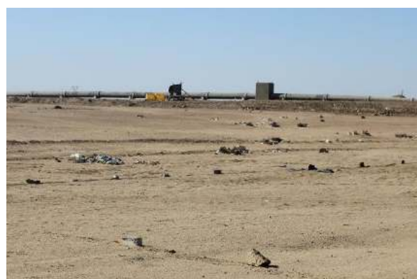
Photo 10. NamWater pipeline cutting across the gravel plains
