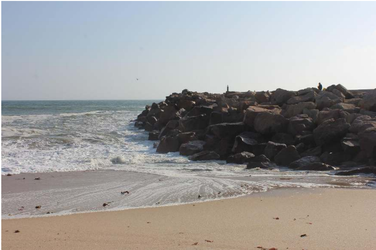
Figure 10. Image showing southern breakwater of harbour and beach, proximal to point of cable landing.
