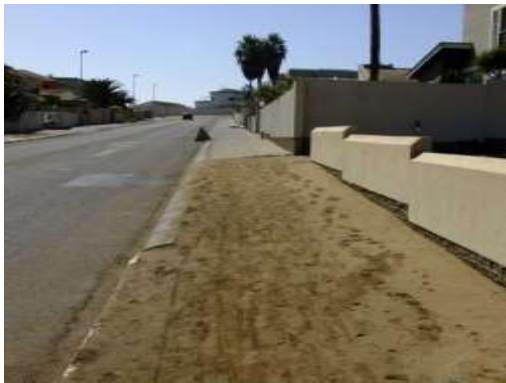
Figure 13: Unpaved pavement with bitumen road
