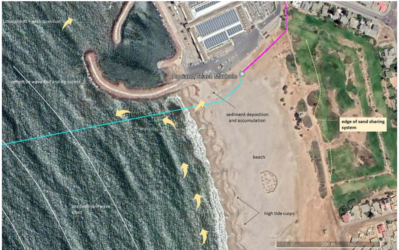
Figure 8. Aerial image of cable landing point showing various coastal processes and features associated with site
