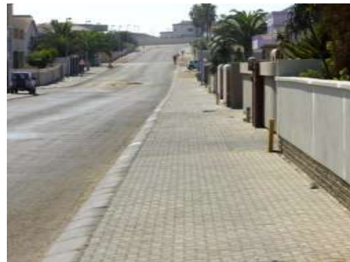
Figure 16: Bitumen surfaced road with interlocked pavement
