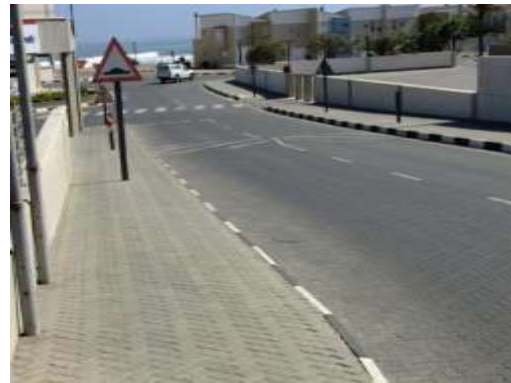
Figure 14: Interlock paving of road and pavement
