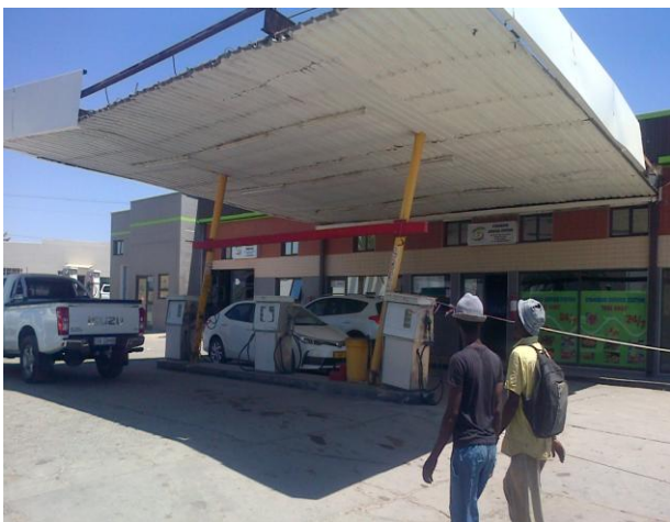
Photo 1. Existing canopy and forecourt
