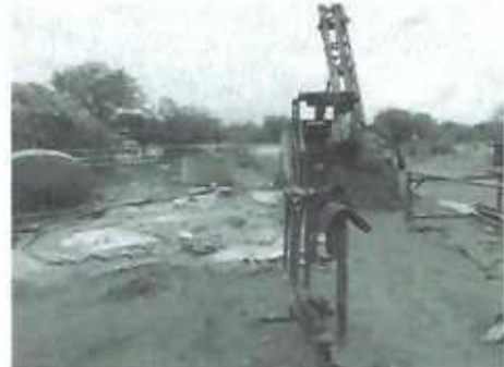
Plastic-lined sumps & Drilling in progress
