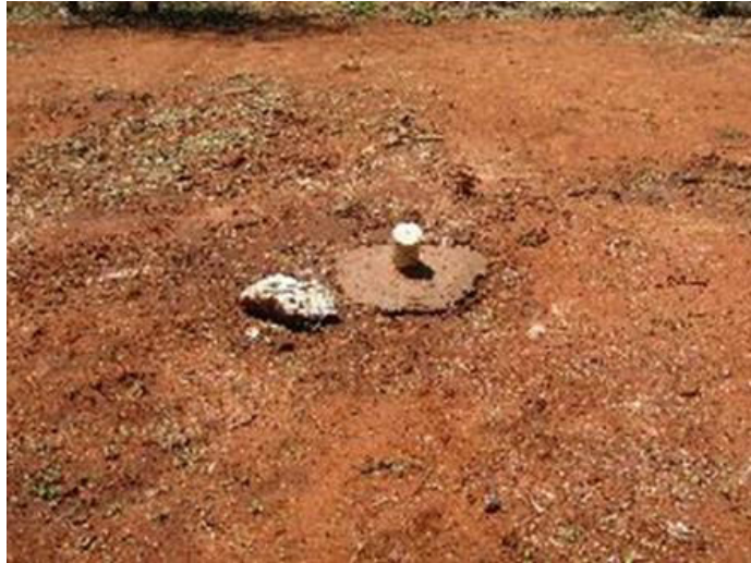
Figure 10 - Cleaned drill-site & capped site
