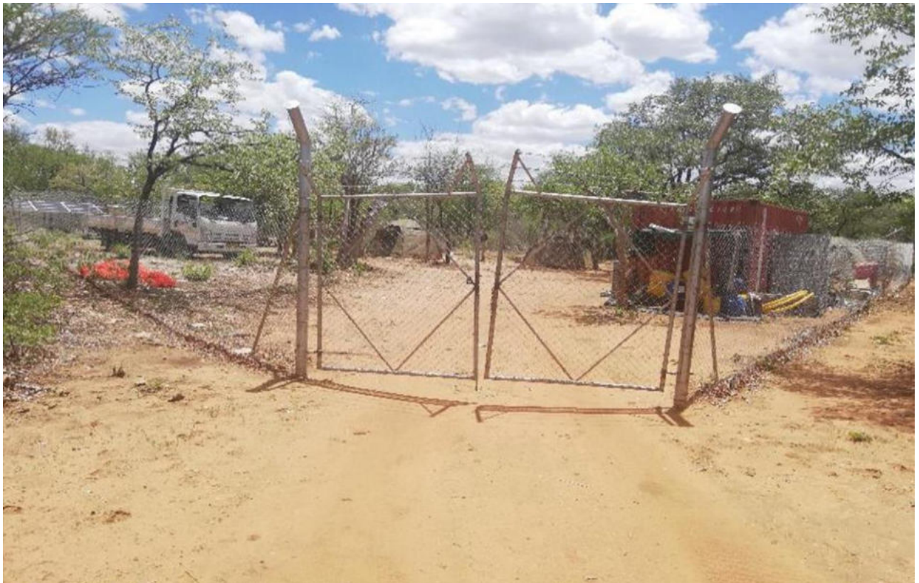
Figure 7 - Fenced camp site with container kitchen, chemical toilets, water borehole, submersible pump and solar panels
