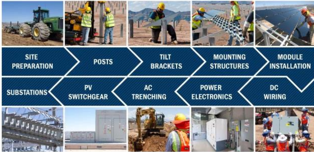
Figure 5: Illustration summarising the construction of a typical Solar PV Power Plant (Source: Solar DAO, 2020)
