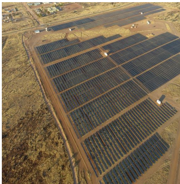
Figure 6: Aerial photograph of existing Gobabis Solar Plant. (Source: Alensy Energy Solutions (Pty) Ltd)
