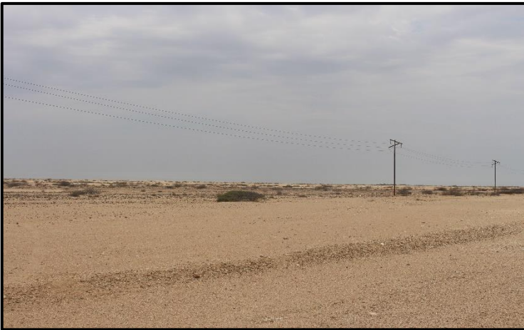
Figure 4: Existing 22KV OHL and cleared servitude
