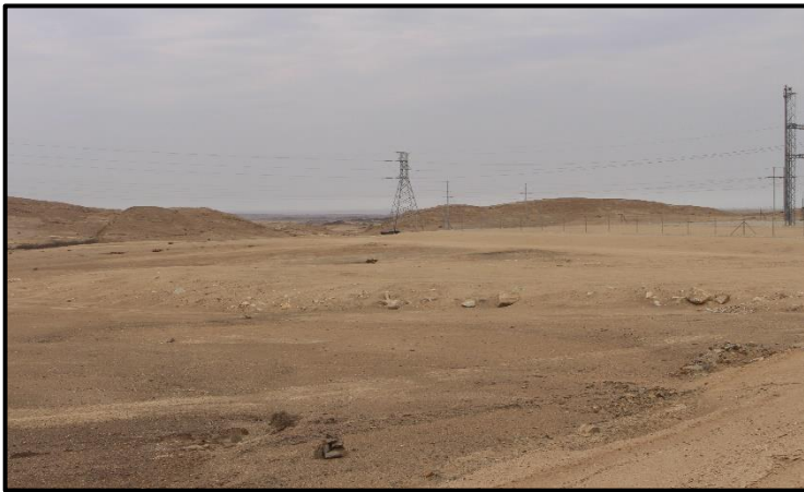
Figure 5: OHL Pylons connecting to Lithops Sub Station
