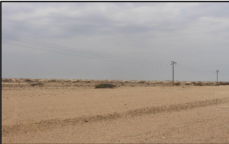
Figure 3: Existing 22KV OHL and cleared servitude
