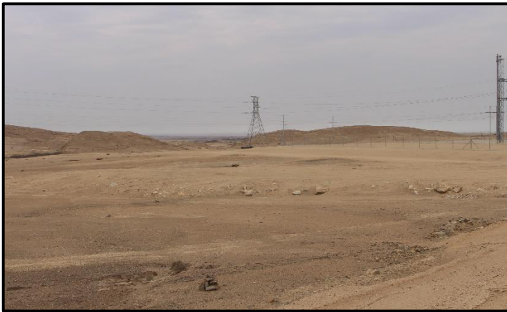
Figure 4: OHL Pylons connecting to Lithops Sub Station
