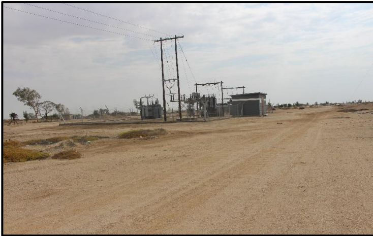
Figure 2: Arandis Sub Station and existing Servitude connecting to B2 Highway.
