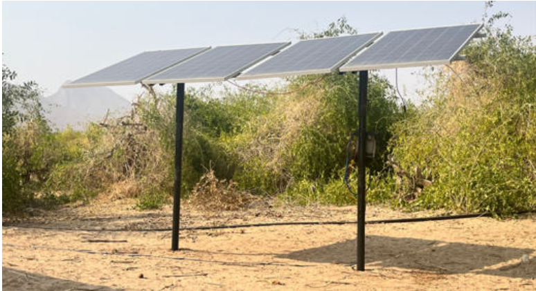
Figure 6. Illustration of solar panel installation
