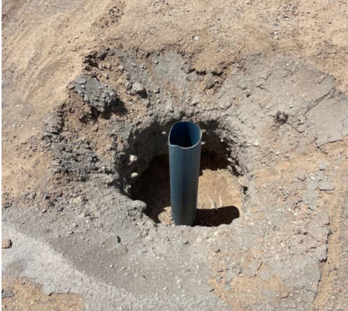
Figure 2 - RC drill hole
