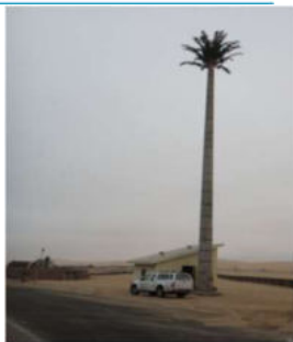
Figure 1: Example of Palmtree Network Tower erected by PowerCom
