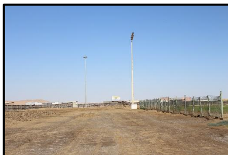
Figure 4: Centre-Existing infrastructure on site
