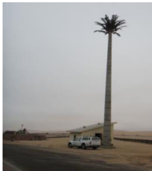
Figure 1: Example of the proposed Palmtree Tower ( https://powercom.na/ )
