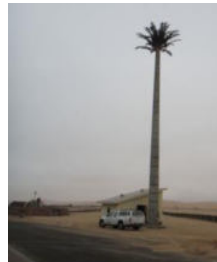
Figure 1: Example of palmtree Network Tower erected by PowerCom
