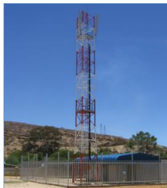
Figure 2: Example of the proposed Lattice Tower ( https://powercom.na/ )
