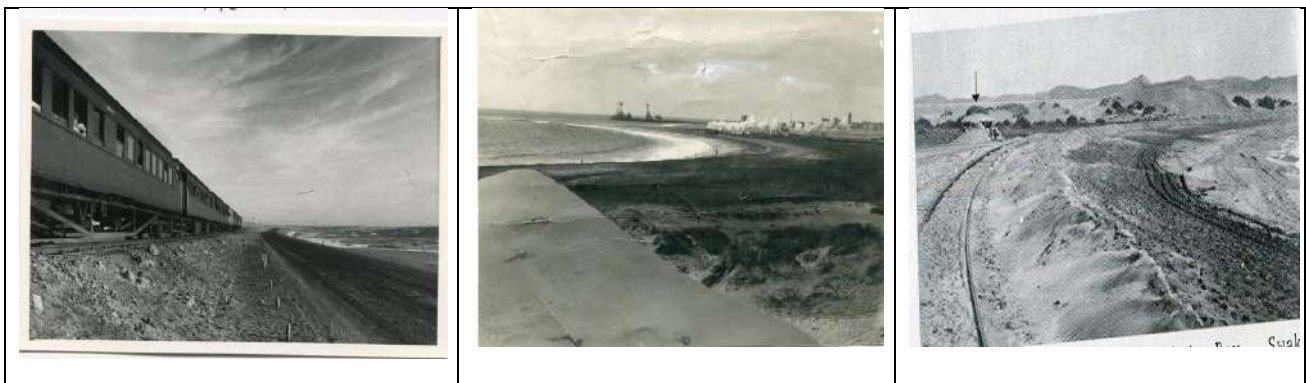
Figure 1.2 Old Railway line photos
