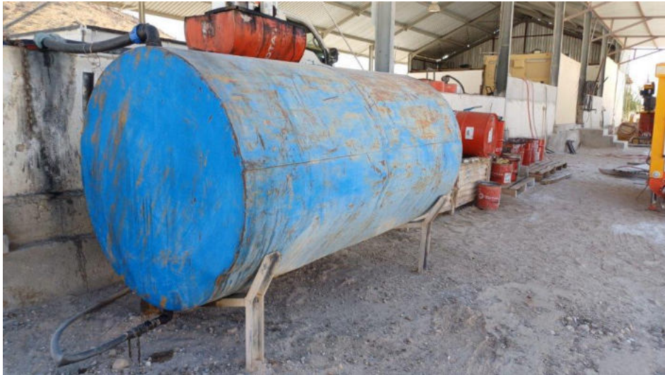
Photo 11 – View of storage tank for used oils and diesel, which is removed by external contractor for reuse.
