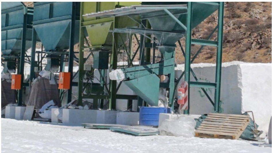
Photo 28 - View of process area which is well maintained and organised.
