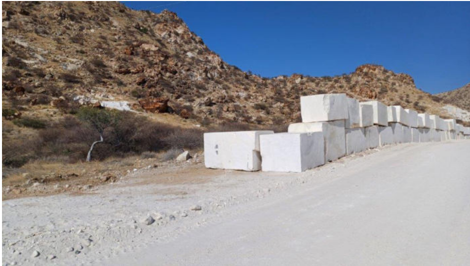
Photo 5 – View of marble wall constructed along the entrance road to the mine to restrict access to the adjacent restricted area (i.e., heritage remains – bushman paintings).
