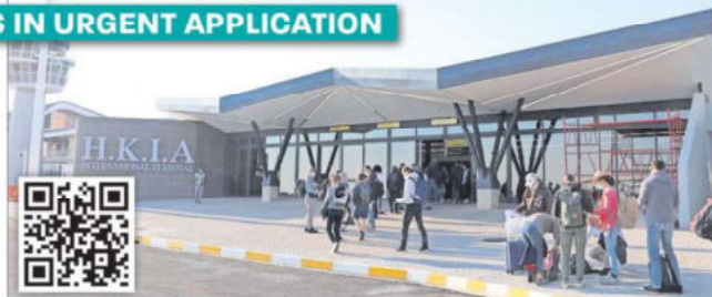
DISMISSED: The Windhoek High Court dismissed Menzies' latest application over ground-handling services at the Hosea Kutako International Airport. PHOTOS: FILE
