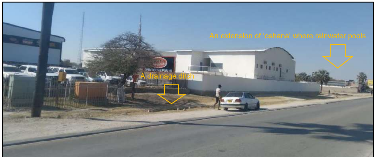
Figure 10: Sections around the hotel where surface water occurs
