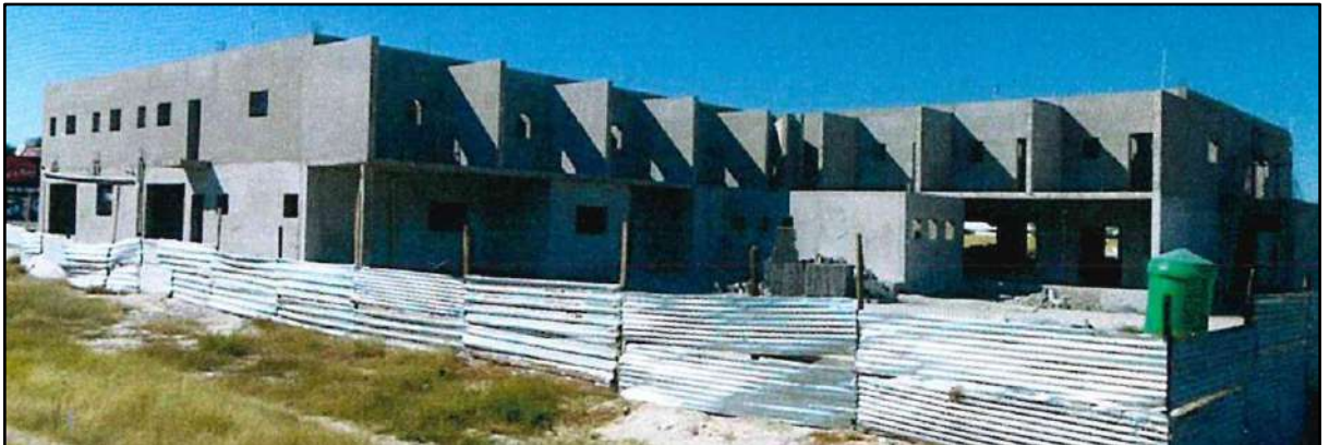
Figure 3: Building Work Halted Due to Covid – 2021
