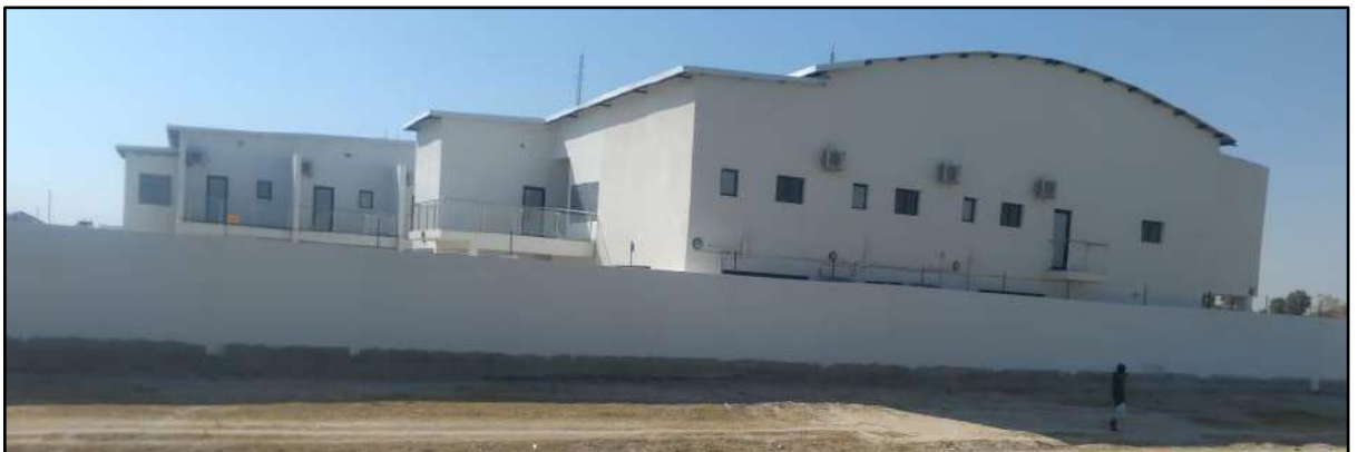
Figure 4: Emirate Hotel nearing completion – June 2023
