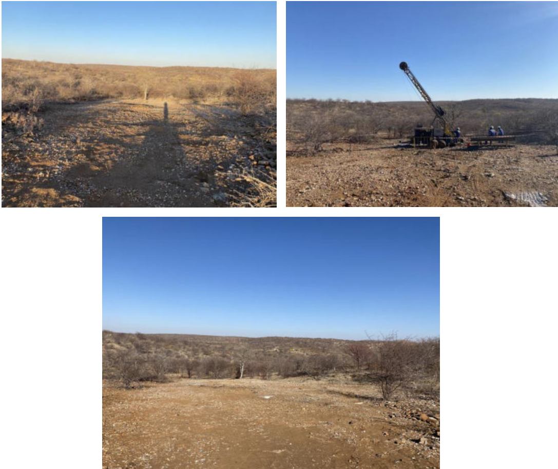
Figure 5 – Images showing diamond drill site LND0005 before, during and after drilling
