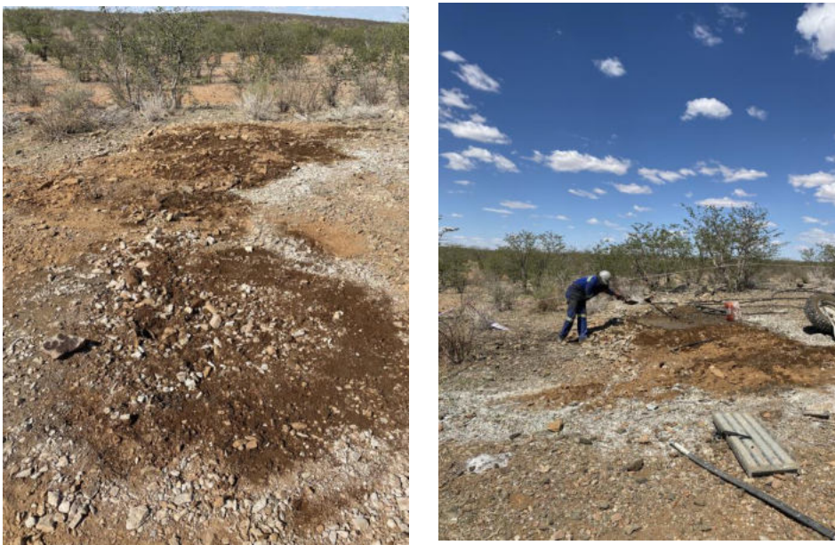
Figure 6 - Rehabilitated drill area and sump rehabilitation at diamond drill site L4D0126.
