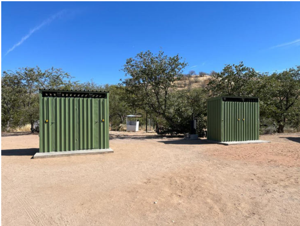
Figure 8 - Toilets and showers constructed in 2022
