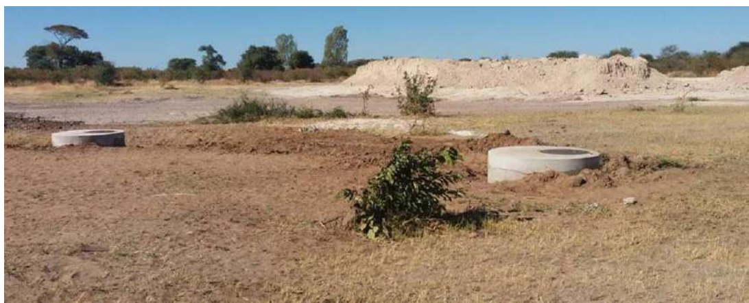
Figure 12: Sewerage Installation underway at another site in Bukalo
