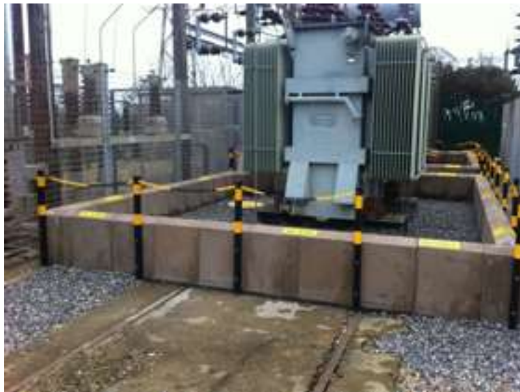
FIGURE 4 - AN IMAGE OF A TRANSFORMER BUDWALL (B2Gold, 2020)
