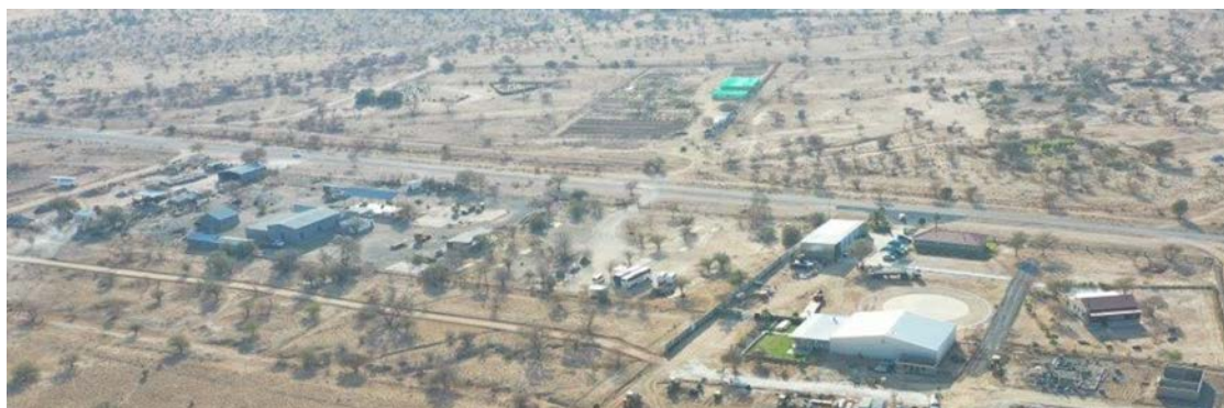
Photo 5.1 – View of build-up industrial like activities & buildings
