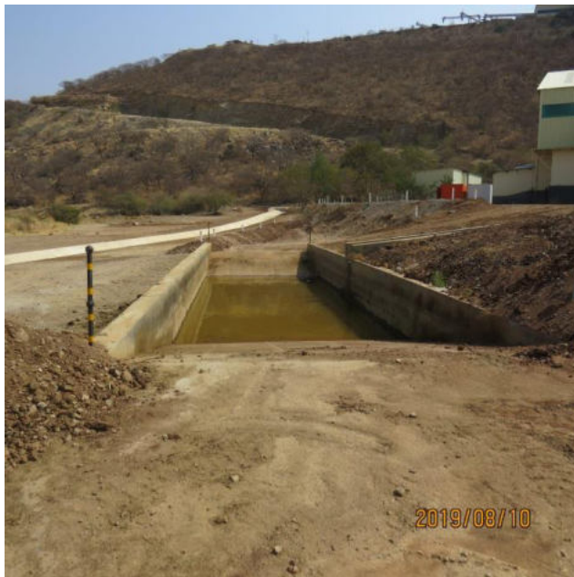
Oil water separator below the wash bay
