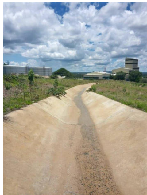
Storm water channel around NTSF
