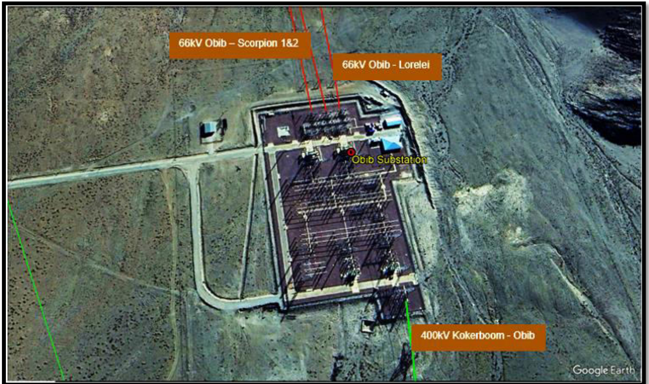
Figure 2: The Obib Substation and associated infrastructures
