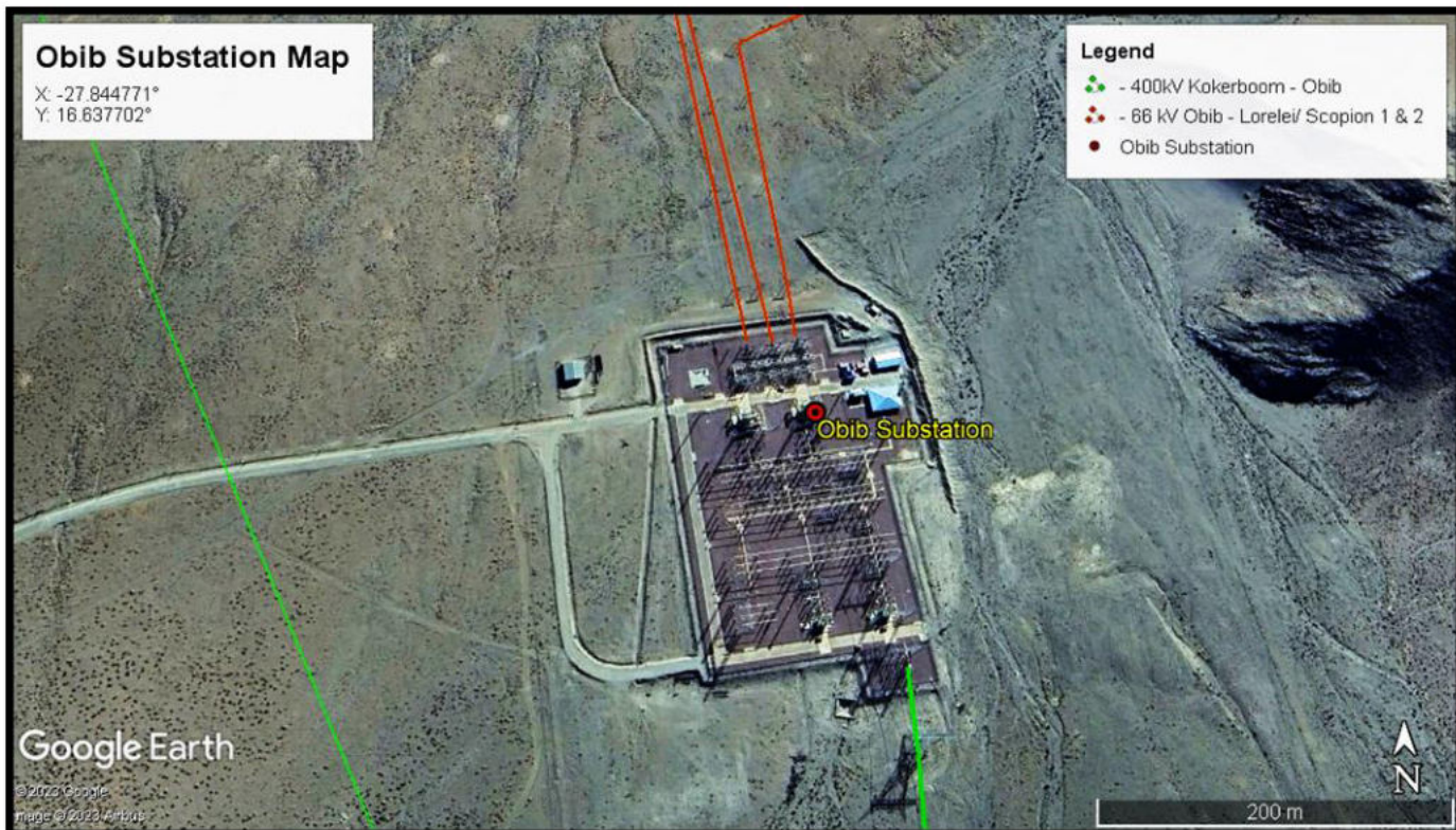
Figure 1: Locality map showing Obib substation
