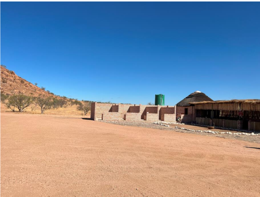
Figure 2.4: The reception and craft stalls that are still under construction.
