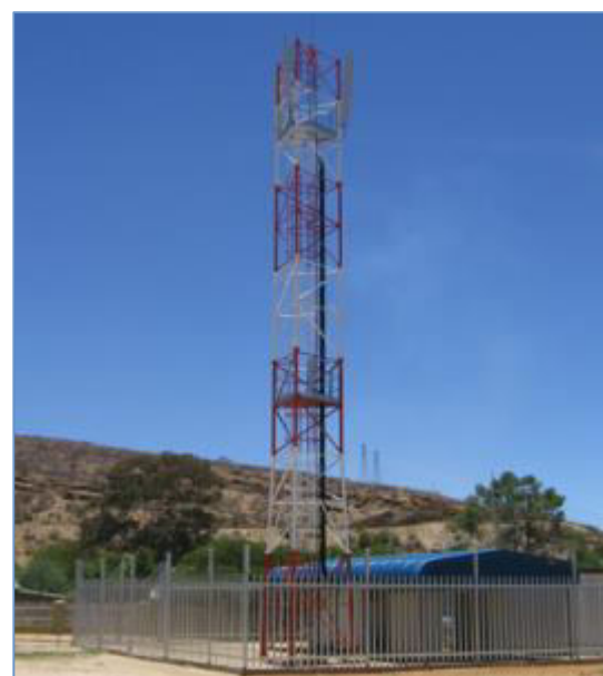
Figure 2: Example of the proposed Lattice Tower ( https://powercom.na/ )
