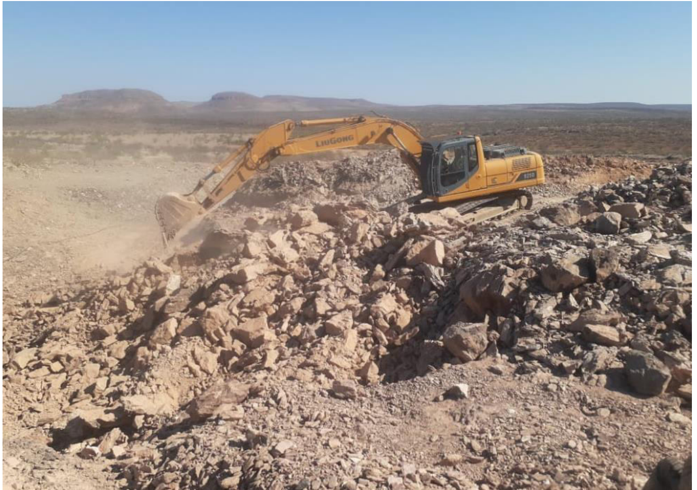
Photo 2, Showing rock samples after blasting
