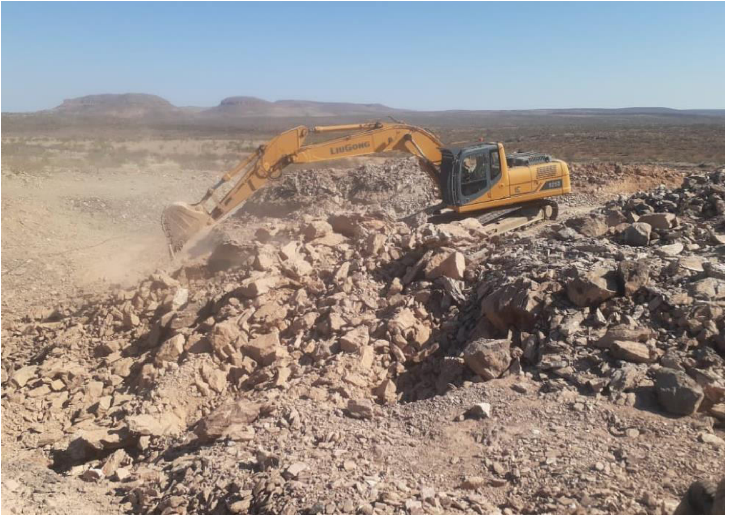
Fig 6 , Showing rock samples after blasting
