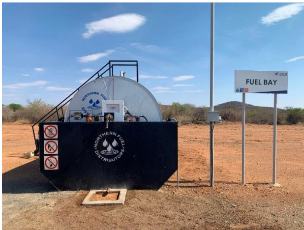
Figure 8. Self bunded fuel storage tank.
