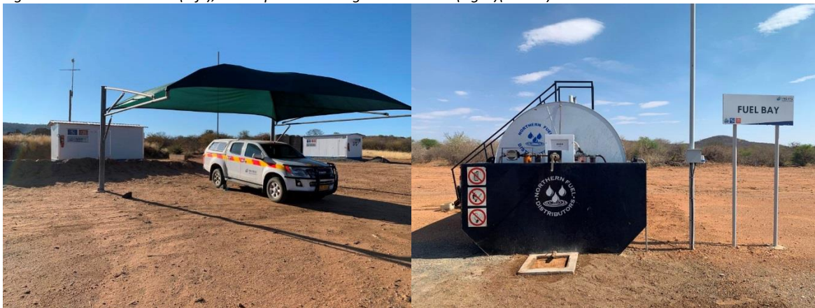
Figure 6. Parking and offices (left), and fuel bay (right)
