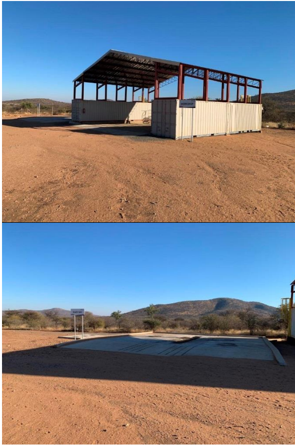
Figure 4 to Figure 6 renders images of these structures. Signage and the general housekeeping is being maintained well.
