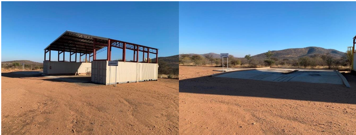
Figure 4. Vehicle workshop (left) and wash bay (right).(6.8.20)
