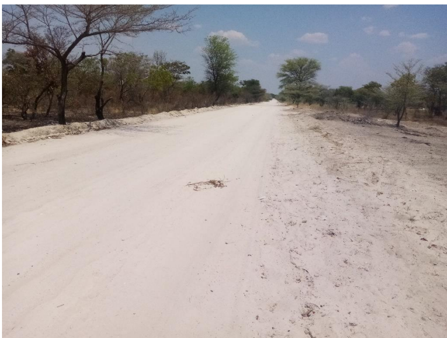
Figure 3: Access road to the project site
