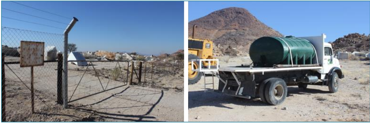
Fig 5: Mine site with the key infrastructure depicted in the background i.e. site fence and entry gate, water supply truck
