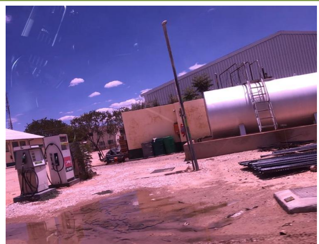
Photo 2. Existing tanks at site
