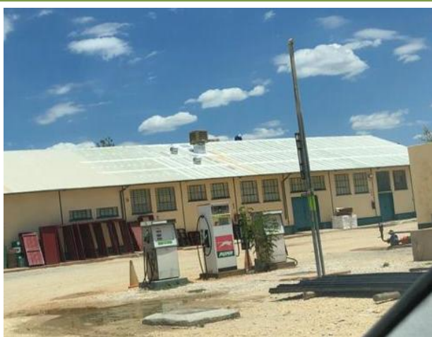
Photo 1. Existing dispensing and vent pipes
