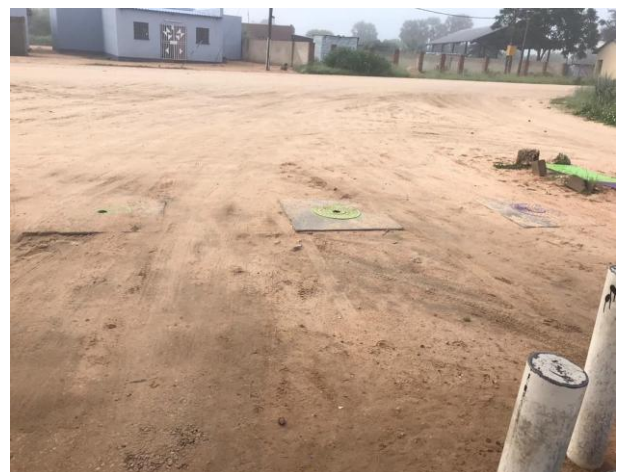
Photo 2. Existing underground storage tanks
