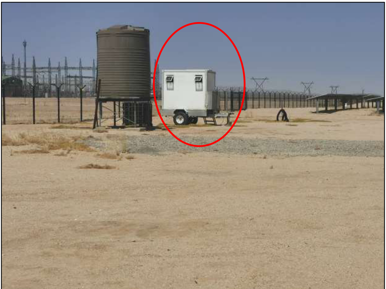
Figure 2-4: The white mobile toilet facility next to the site water storage tank at the PV Plant entrance
