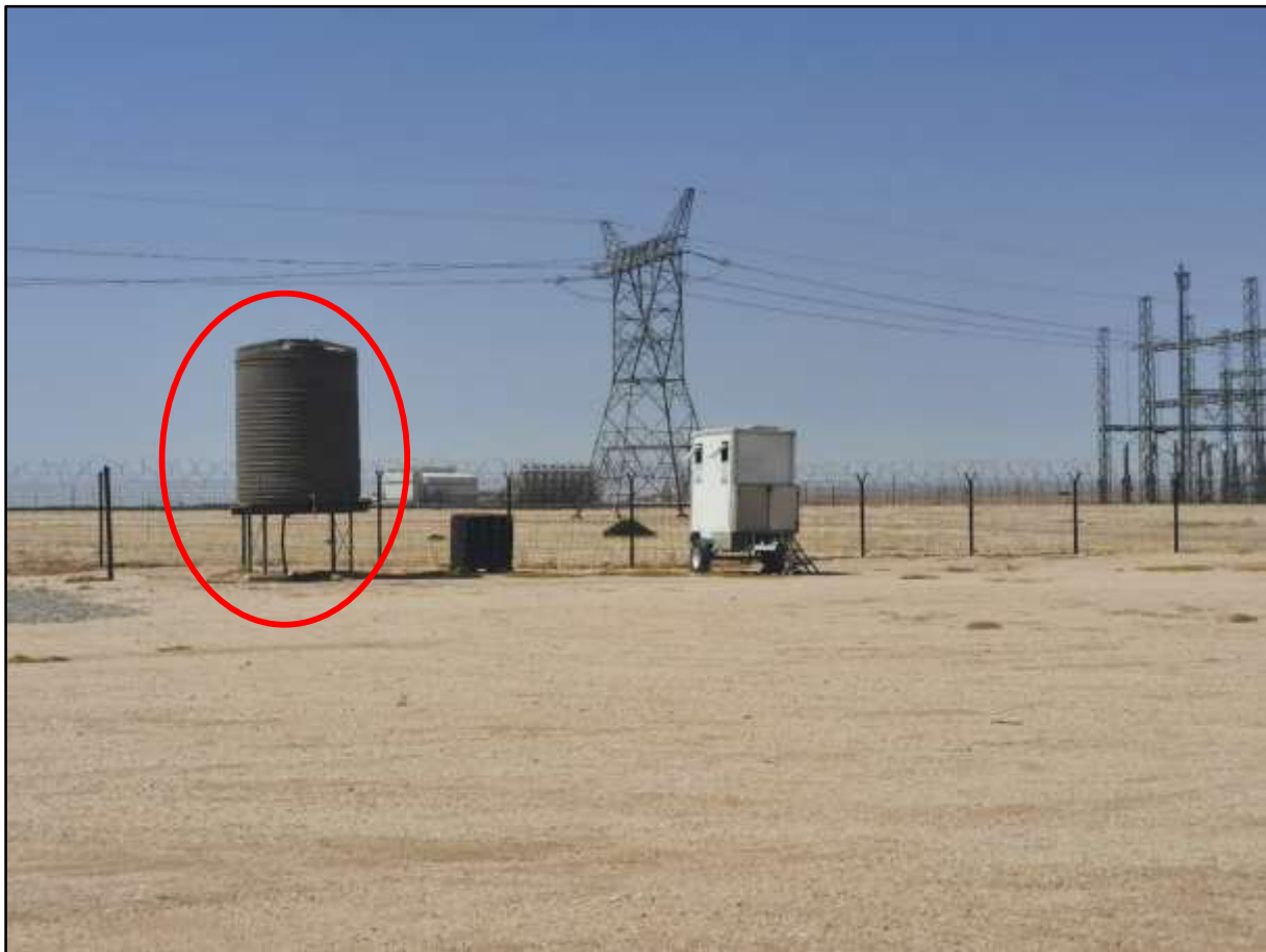
Figure 2-3: The water storage tank (next to the white mobile toilet facility) near the PV Plant entrance
