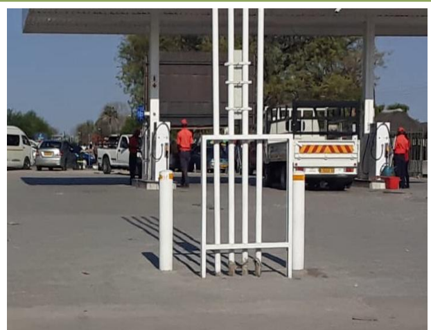
Photo 2. Existing canopy and vent pipes
