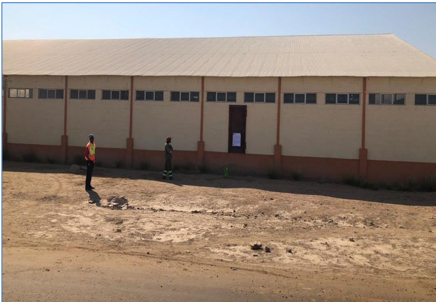
Figure 5: Building on Project Site
