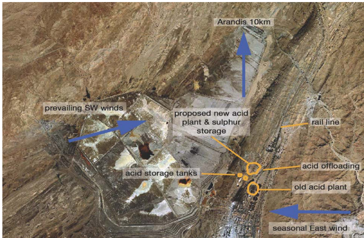
Figure 10: Overlain on an aerial photograph, the proposed location of the new RUL acid plant relative to the old acid plant and other related sulphuric acid producing infrastructure (source: RUL public participation material, 2007)
