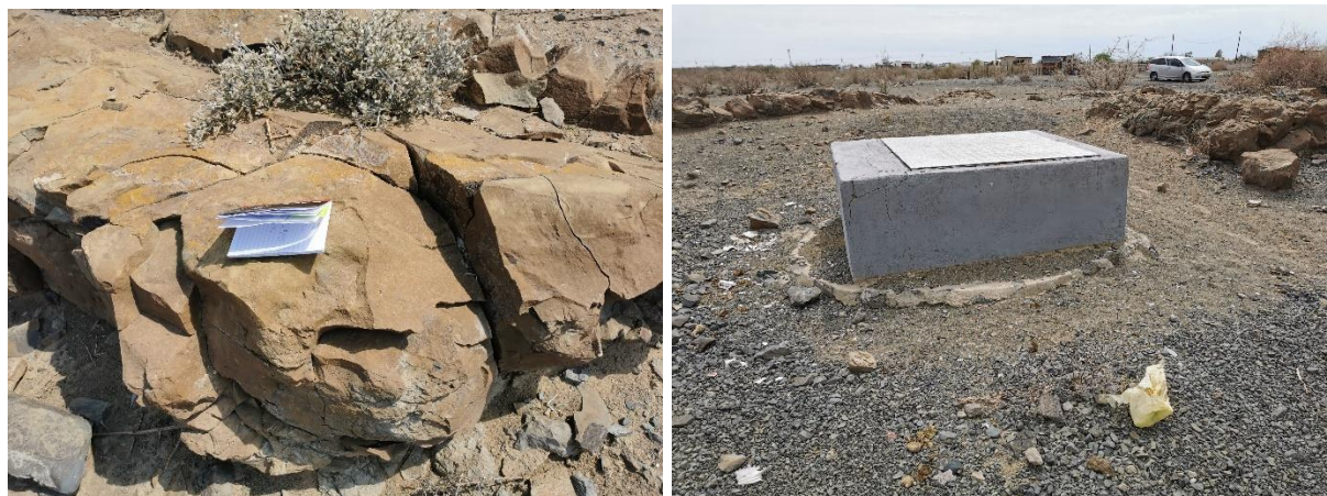
Figure 15: Shale outcrops at the ponds' site area and the manhole within proximity of the ponds
