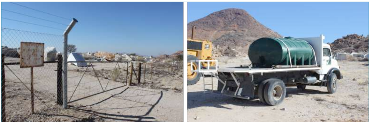
Fig 12: Mine site with the key infrastucture depicted in the background i.e. site fence and entry gate, water supply truck
