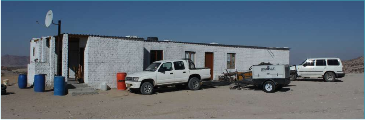
Fig 13: Shows the Staff Accommodation and Current Office Facility (including ablutions), in foreground is the feed collection (light vehicle and compressor equipment)
