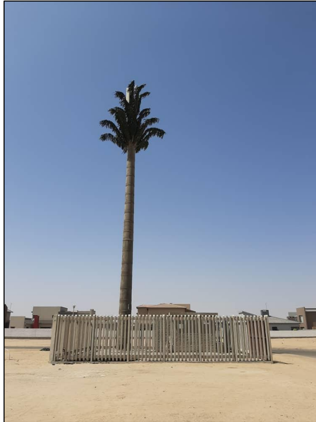
Figure 2-3 : Tower erected on Erf 5361, Ocean View
