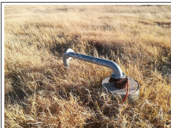
Photo 4-14 Typical borehole installation on Farm Okasodana
