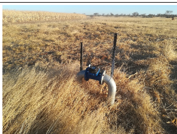
Photo 4-15. Typical flowmeter installation on the Farm Evare
