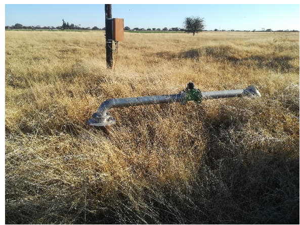
Photo 4-8. Power and water supply infrastructure on the Farm Evare
