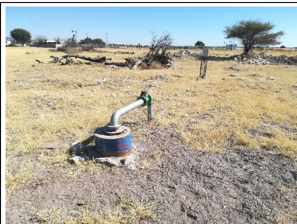
Photo 4-18 Typical borehole installation on Rika No. 266 (Portion 1)
