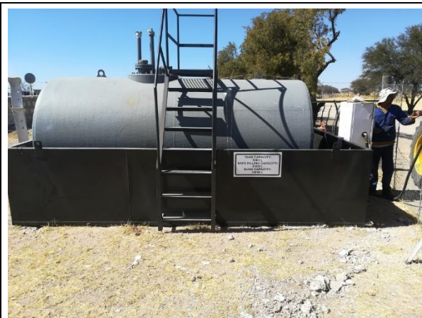
Photo 4-22. Diesel tank (9 m 3 )
