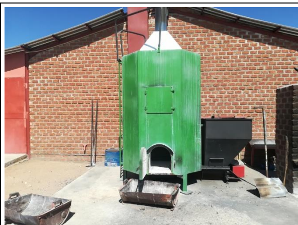
Photo 4-5. Drier room furnace
