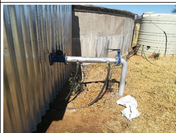
Photo 4-20. Flow meter from the fertiliser mixing tank on the farm Bosville
