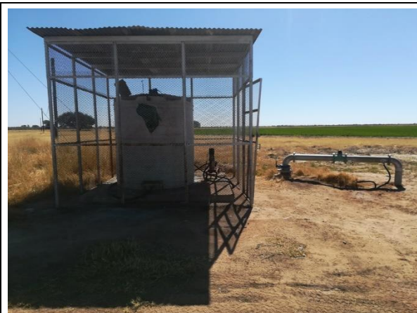
Photo 4-3. Fertilizer mixing tank
