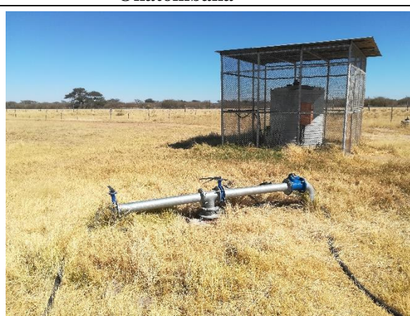
Photo 4-21. Borehole with flow meter and fertiliser mixer on the Farm Okatombaka
