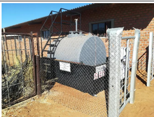
Photo 4-23. Diesel tank (4.9 m 3 )
