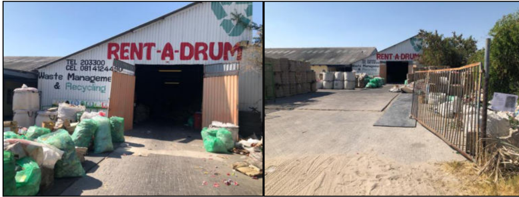
Figure 3: Entrance to the operational area
