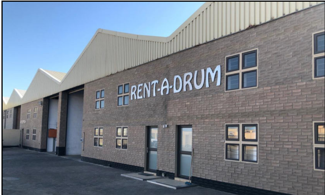
Figure 3: Main building on site
